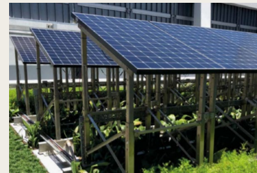
Figure 7: dual-level roof of integrated solar PV and green roof
